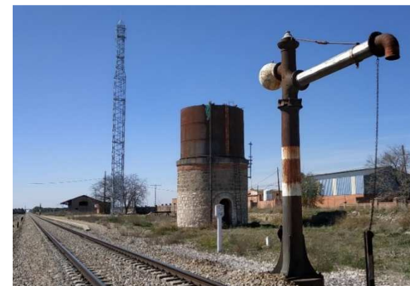
□ Installation of GSM-R railway towers.
