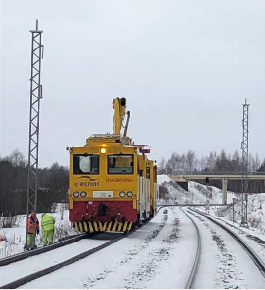
□ Electrification project of the high-speed railway corridor in Lithuania.
