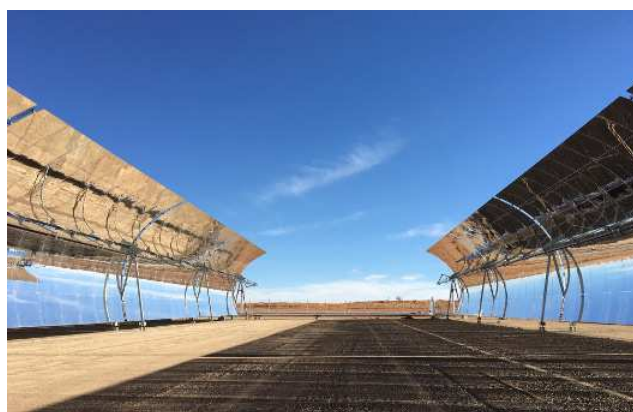
□ Parabolic trough solar thermal plant for Xina Solar One (Northern Cape, South Africa).
