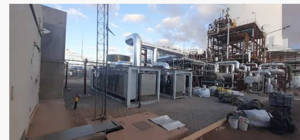
□ Khi Solar One booster heater, an item not included in the original design of the plant which was included in the Action Plan.
