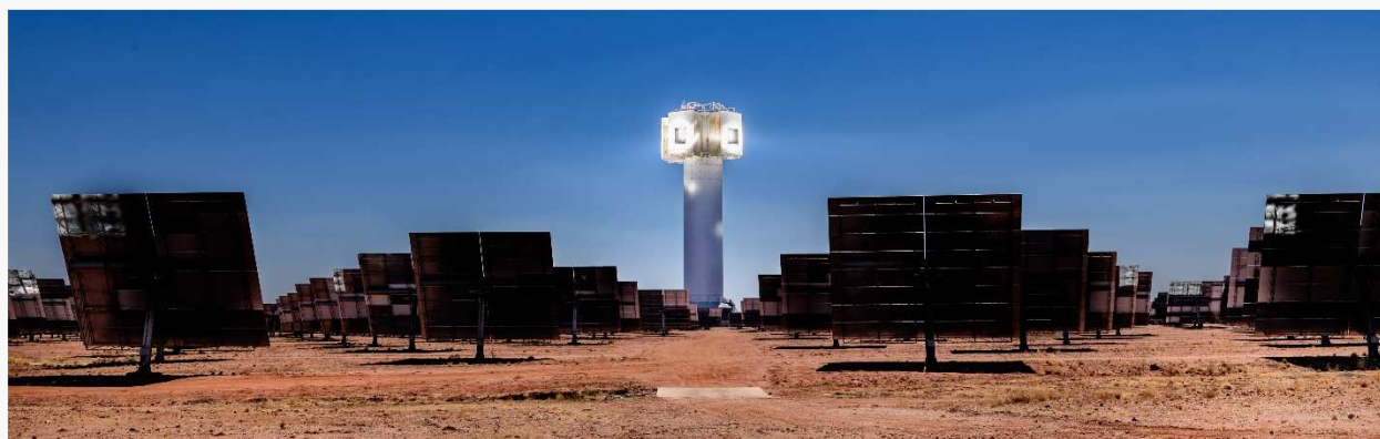
□ Khi Solar One thermal solar power station in operation.
