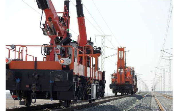
□ Maintenance work on the electrification infrastructure of the high-speed train Mecca-Medina.
