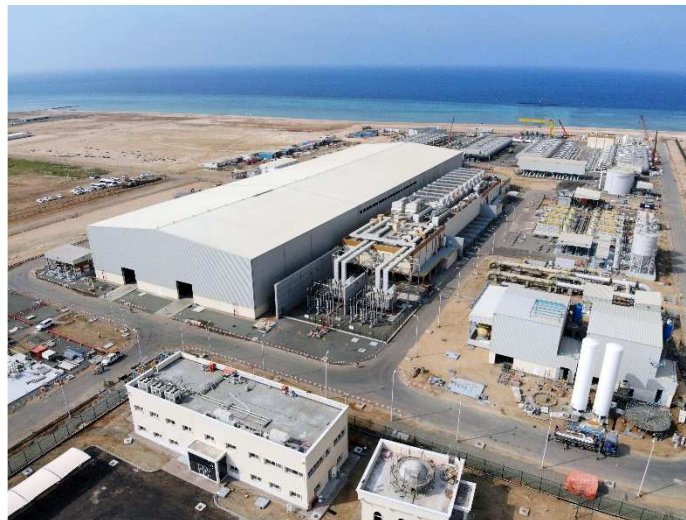
□ Reverse osmosis desalination plant in Saudi Arabia.
