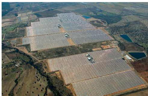
□ Extremadura Solar Platform solar thermal parabolic trough collector power plant (Logrosán, Cáceres, Spain).
