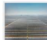
1/3/23 Abengoa celebrates 3 years without a Lost Time Work Accident at Noor Energy I sola...
