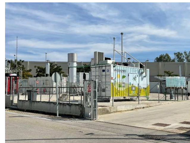
□ Grasshopper, pilot plant for producing electricity from hydrogen.
