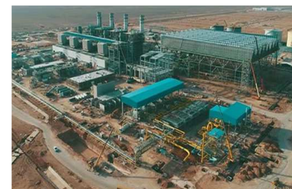
□ Hybrid solar-gas plant in Hassi R'Mel (Hassi R'Mel, Algeria).
