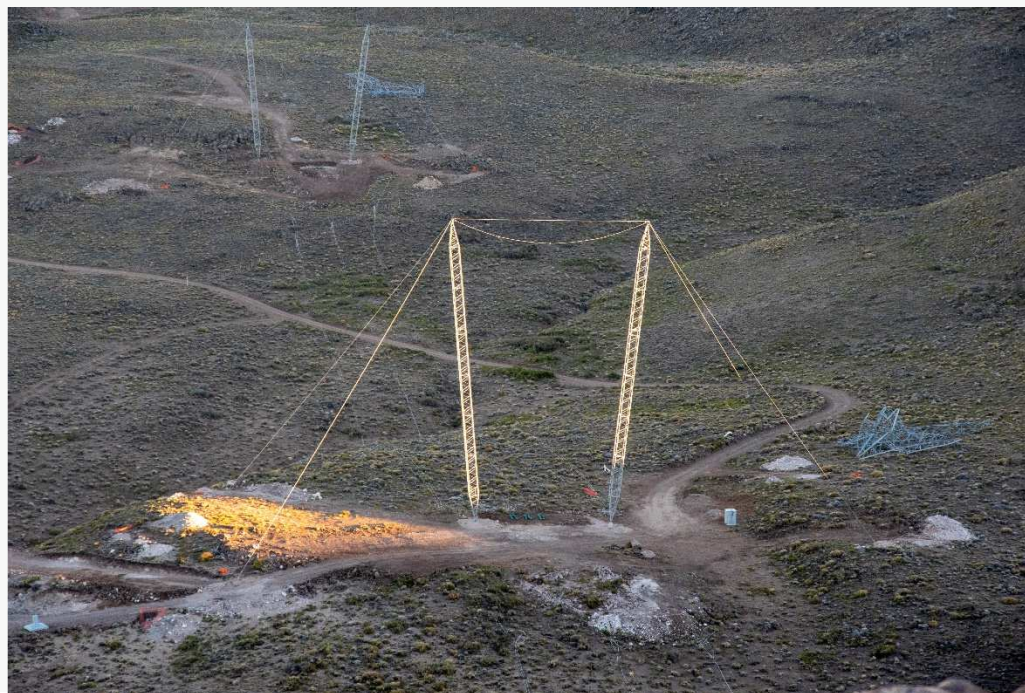
□ Repair work on the 330kV Futaleufú line: Situation afterwards.
