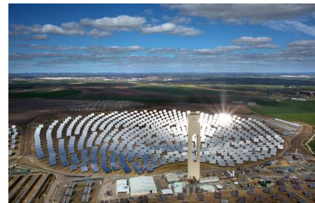
□ Solar thermal tower for the Solucar Platform (Seville, Spain).
