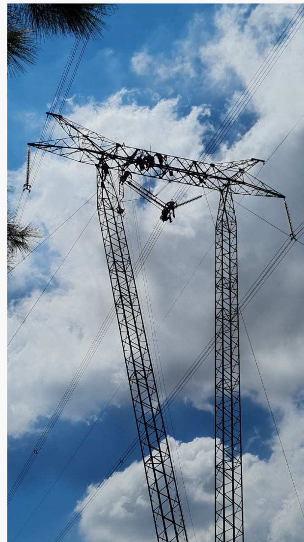
□ Maintenance work on transmission lines in Brazil.
