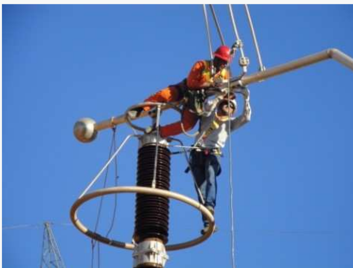
□ Maintenance work on transmission lines in Brazil.
