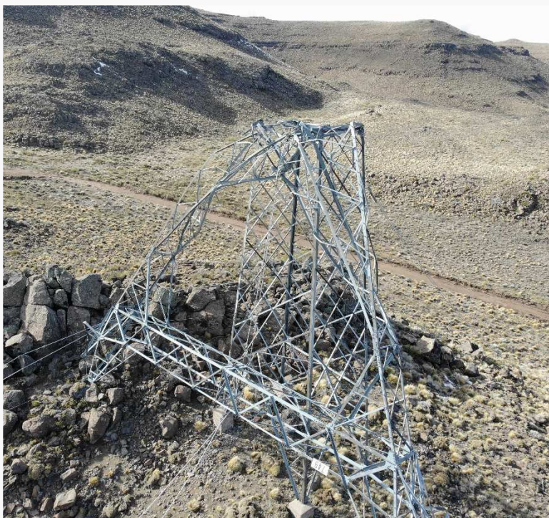
□ Repair work on the 330kV Futaleufú line: Previous situation.
