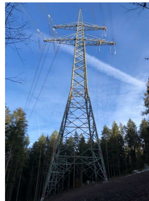
□ Manufacture of metal structures for Ostbayernring Tennet project in Germany.
