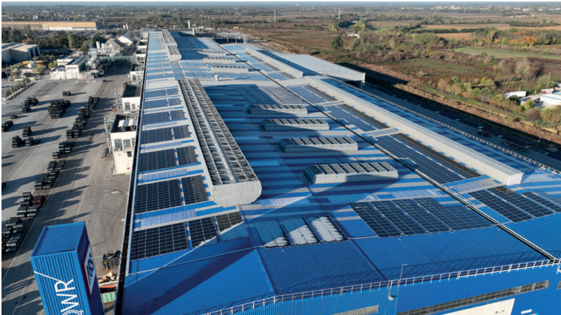
Photo: The photovoltaic plant in Saturno line.
