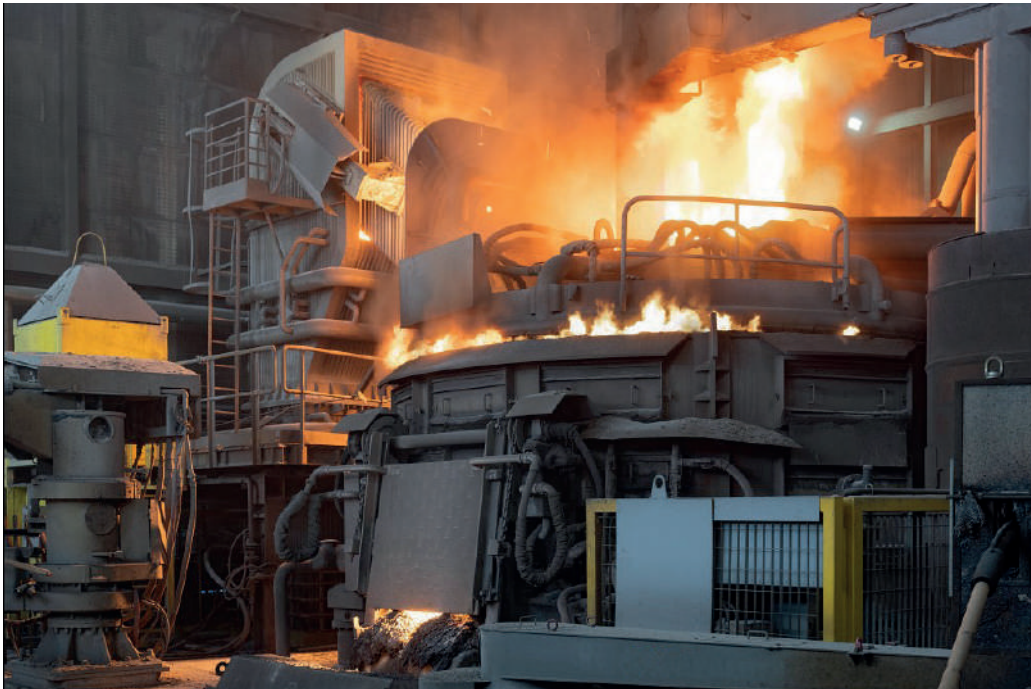
Photo: Furnace at the ABS Sisak production plant (Croatia).
