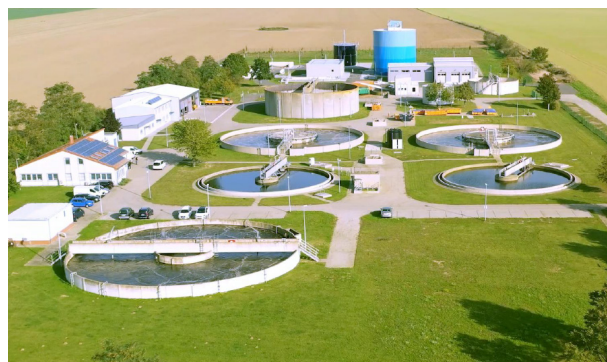
Figure 8: Wastewater treatment plant in Roskow, which was equipped with new technology by the Aerzen Group in 2024
