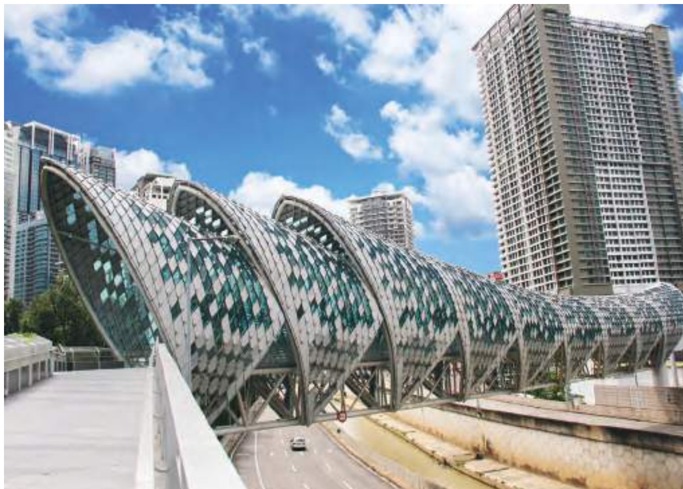
Saloma Link Bridge connecting Kampung Bharu to KLCC in the heart of Kuala Lumpur.
