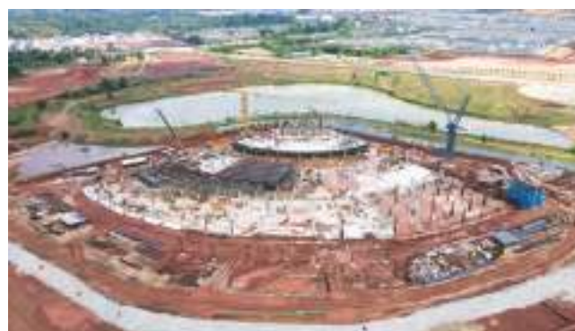
On going project at The Masjid Bandaraya KotaSAS.
