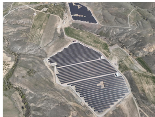
AISIN TURKIYE SOLAR POWER PLANT
