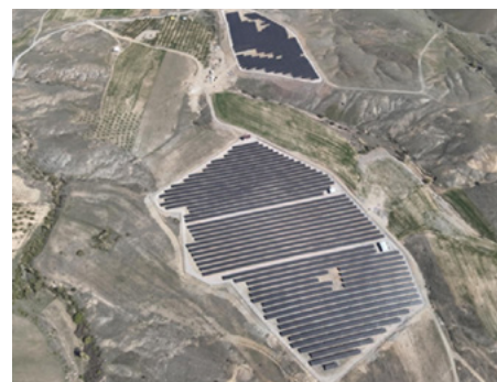
AISIN TURKIYE SOLAR POWER PLANT
