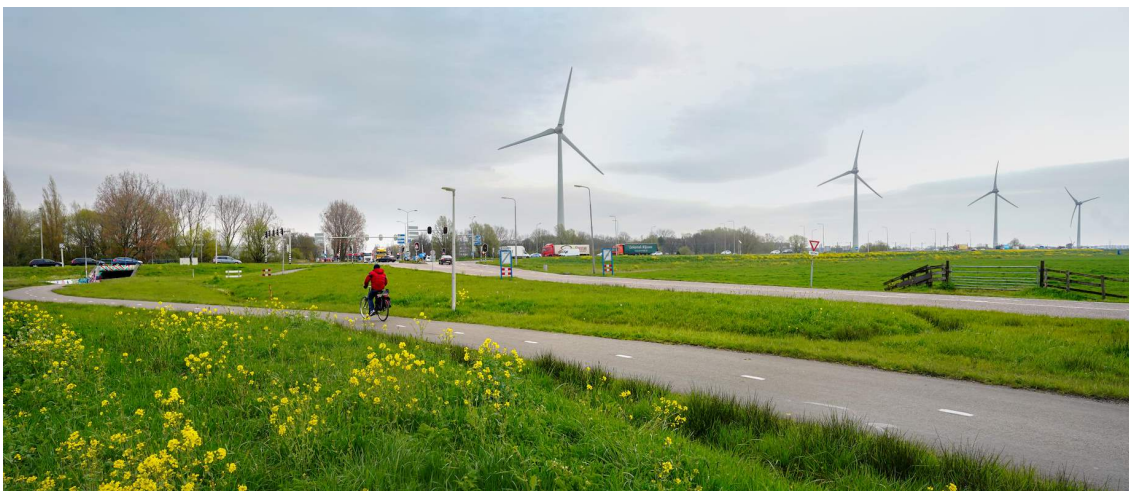
Our expansions, upgrades and modifications make improved sustainability and development in the Netherlands possible.
