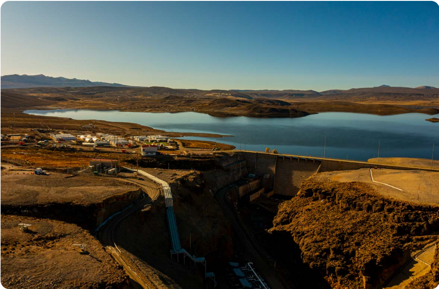
The Vizcachas dam, which we built as part of the Quellaveco project, provides water to the mine, as well as to local communities and agriculture.
