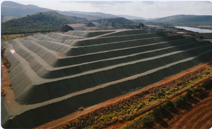
At our Barro Alto and Codemin operations, existing stockpiles of mineral waste will sequester atmospheric carbon and benefit Brazilian agriculture.
