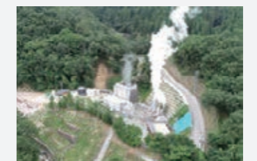
The first geothermal power plant has already started commercial operations.
