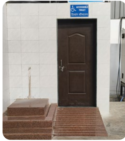
Washroom for specially-abled persons @ APAR Khatalwada Cable Plant
