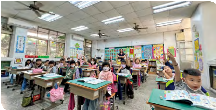
Campus LED Installation Projects (Zhangxing Elementary School)
