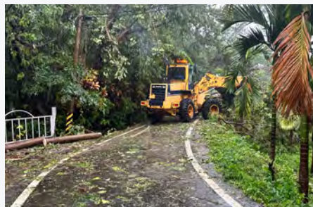
Post-Storm Assistance in Recovery Efforts
