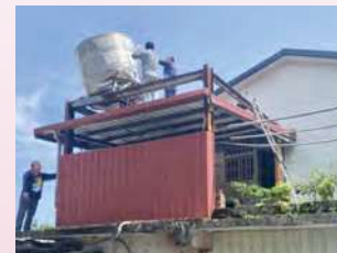
Subsidies for water tank replacement and repairs, and assistance with slope restoration works
