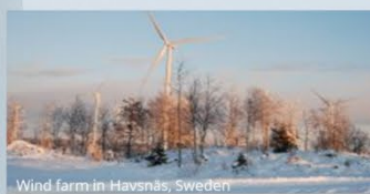
Wind farm in Havsnäs, Sweden
