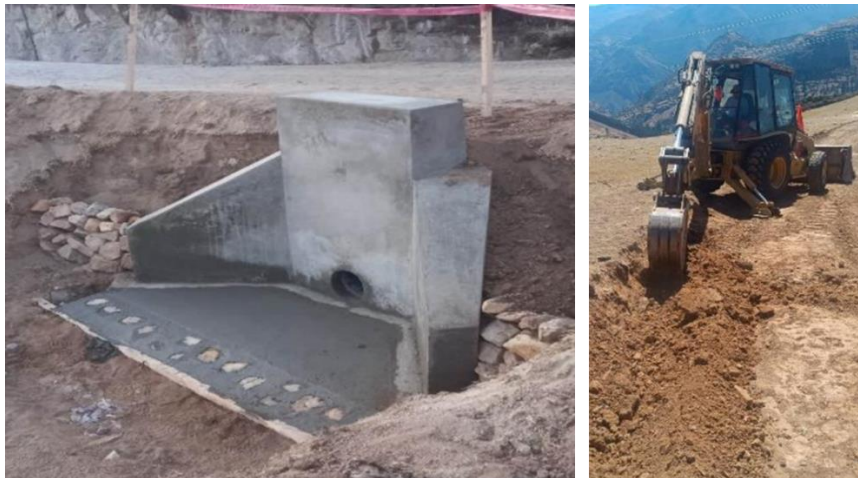
Construction and maintenance of roads
