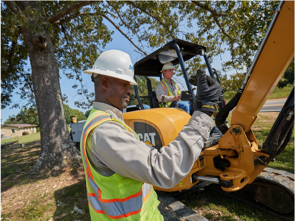
Jack, Senior Service Technician, and Tyler, Senior Construction Operator, work with local Mississippi contractors to provide natural gas service to new customers in the Starkville area.
