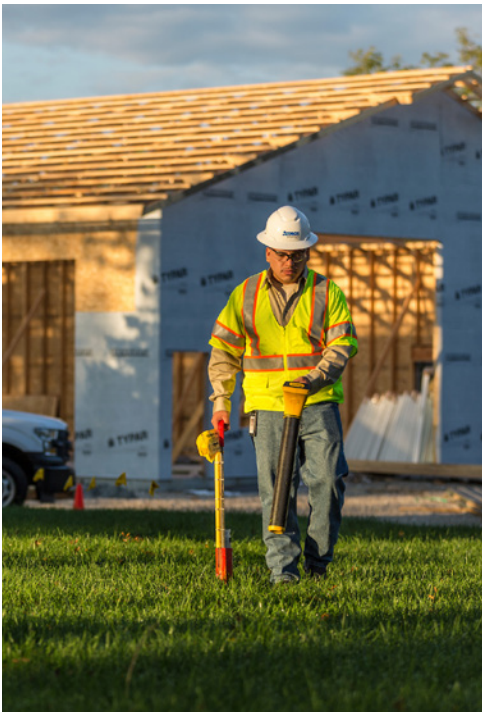
Gerson, a Senior Utility Technician in Kansas, locates and marks underground natural gas pipelines with yellow temporary paint to ensure safe digging.
