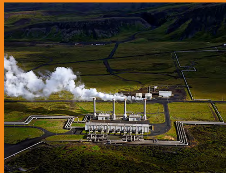
Geothermal power plants help us rewrite The Energy Equation™
