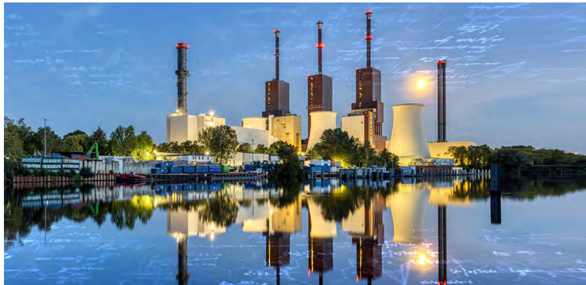
Combined heat and power plant, Berlin, Germany
