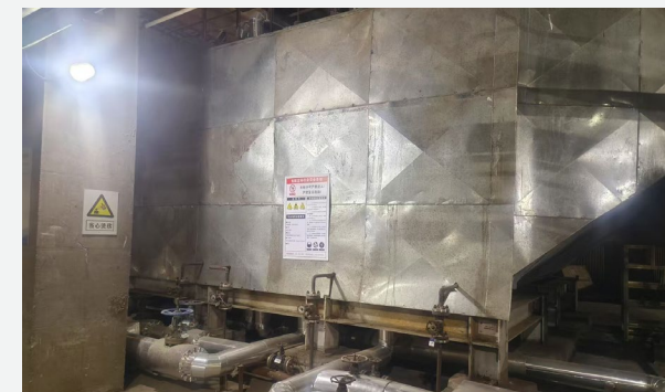
Site for reducing wind temperature in Gaoantun
