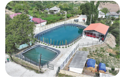
Image: Development of a reservoir and filtration facility in Avaran, Azerbaijan
