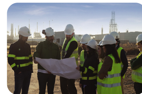
Image: Construction has begun on the green hydrogen project at our Castellón refinery, Spain
