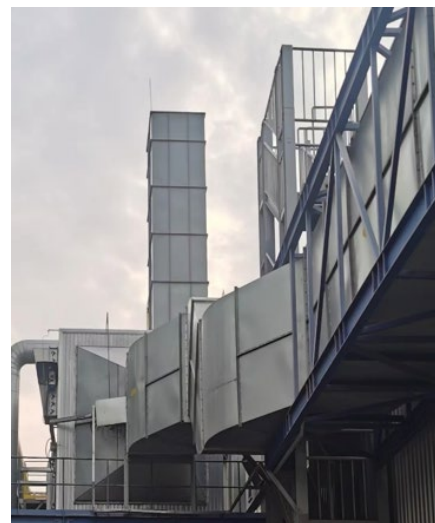
Brother Machinery Xian Co., Ltd.: VOC treatment system
