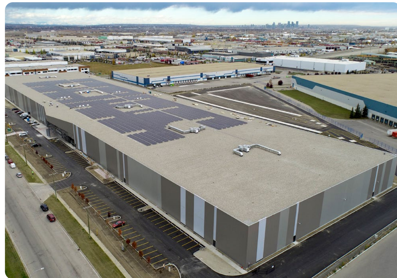
Solar panels on the roof of CT REIT's net zero distribution centre – Calgary, Alberta
