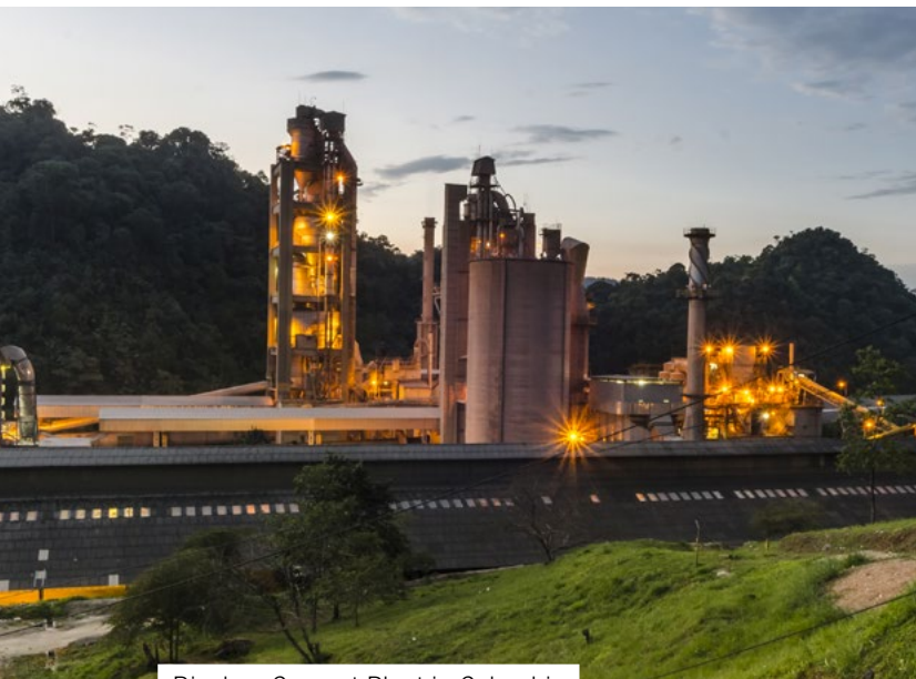
Rioclaro Cement Plant in Colombia
