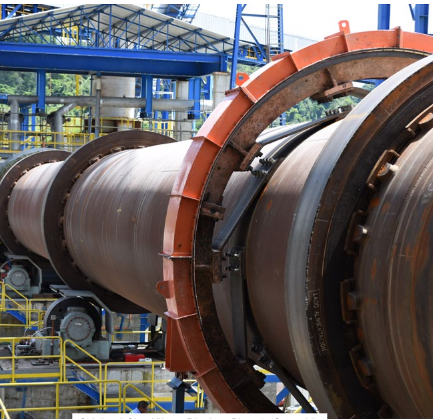
Calcined Clay Kiln at Rioclaro Plant in Colombia
