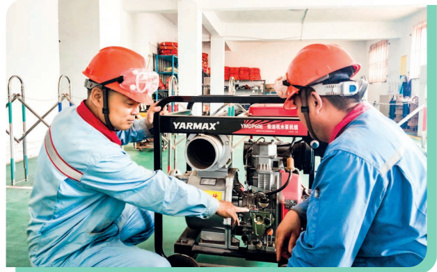
Inspecting Flood Discharge Facilities
