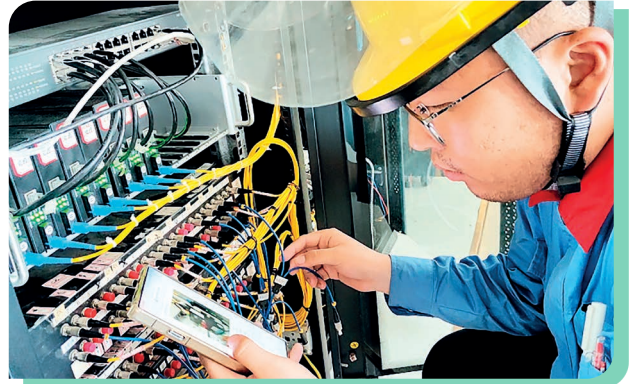
Application of AI Technology Supports Frontline Maintenance Work
