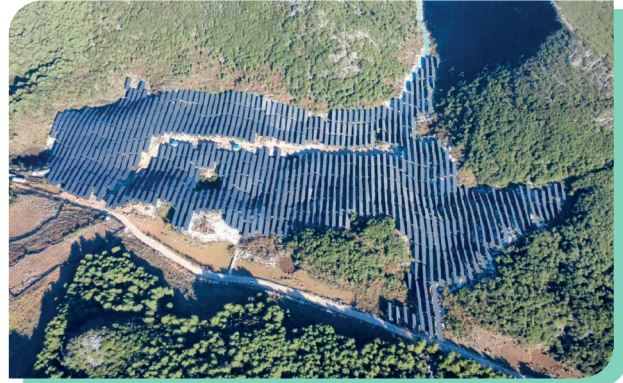
Kongzhaopu Photovoltaic Power Station in Luxi County, Yunnan
