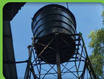
Rain Water Harvesting
