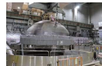
Scene of the removal of the reactor pressure vessel upper head
