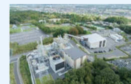
Minokamo Biomass Power Plant
