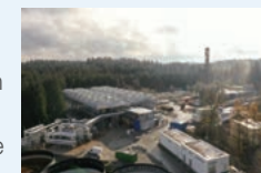
Provision by Eavor Technologies
