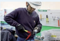
Service drop line dismantling work
