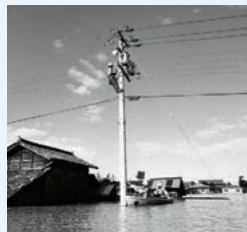
Restored distribution line after Typhoon Isewan (1959)
