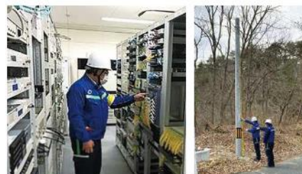
An inspection in progress
