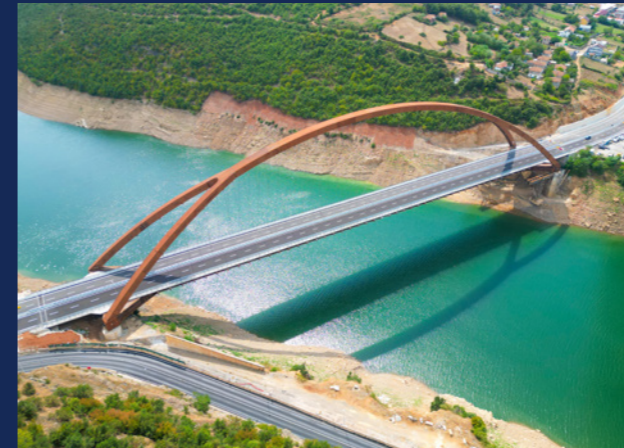
Drini Bridge, Albania.
