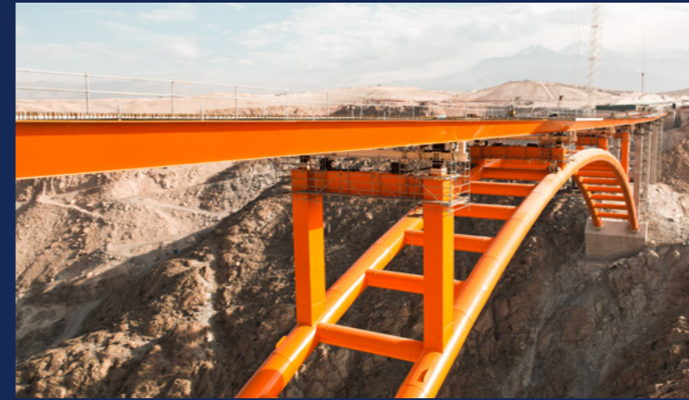
La Joya Bridge, Peru
