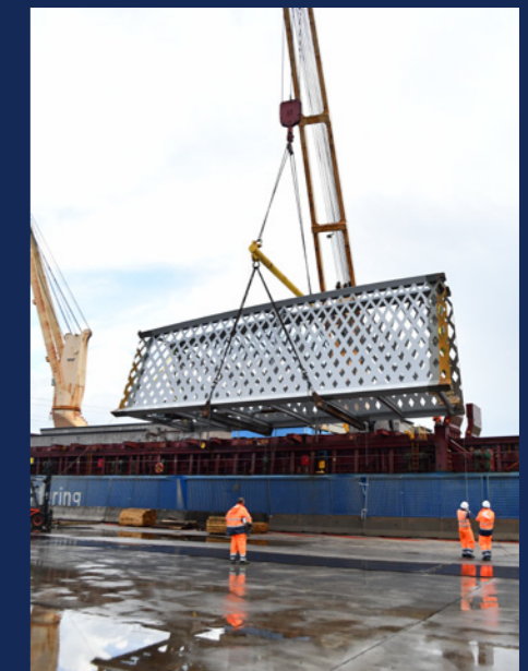
Buffalo Bridge, USA
