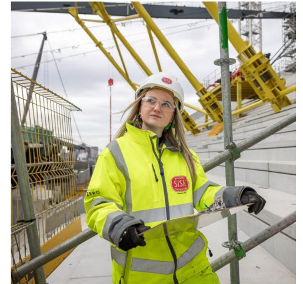
Apprentices with Sisk, working on Manchester City's north stand
