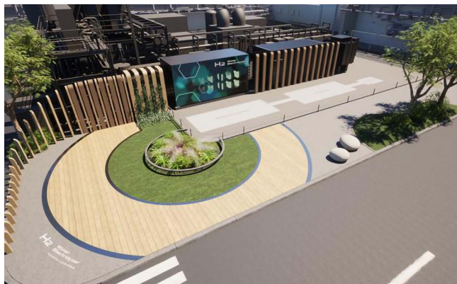
The completed Hydrogen Park at Toyota's Honsha Plant
