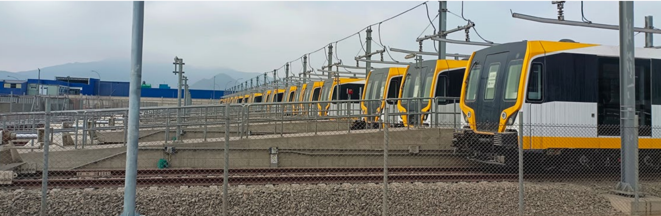
Maintenance of the underground line Metro in Lima (Peru). ▼
