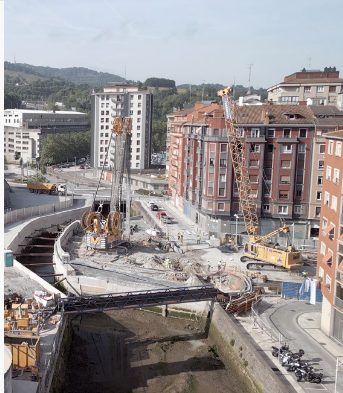
Work on the Altza-Galtzaraborda section of the Donostia Metro (Spain).
