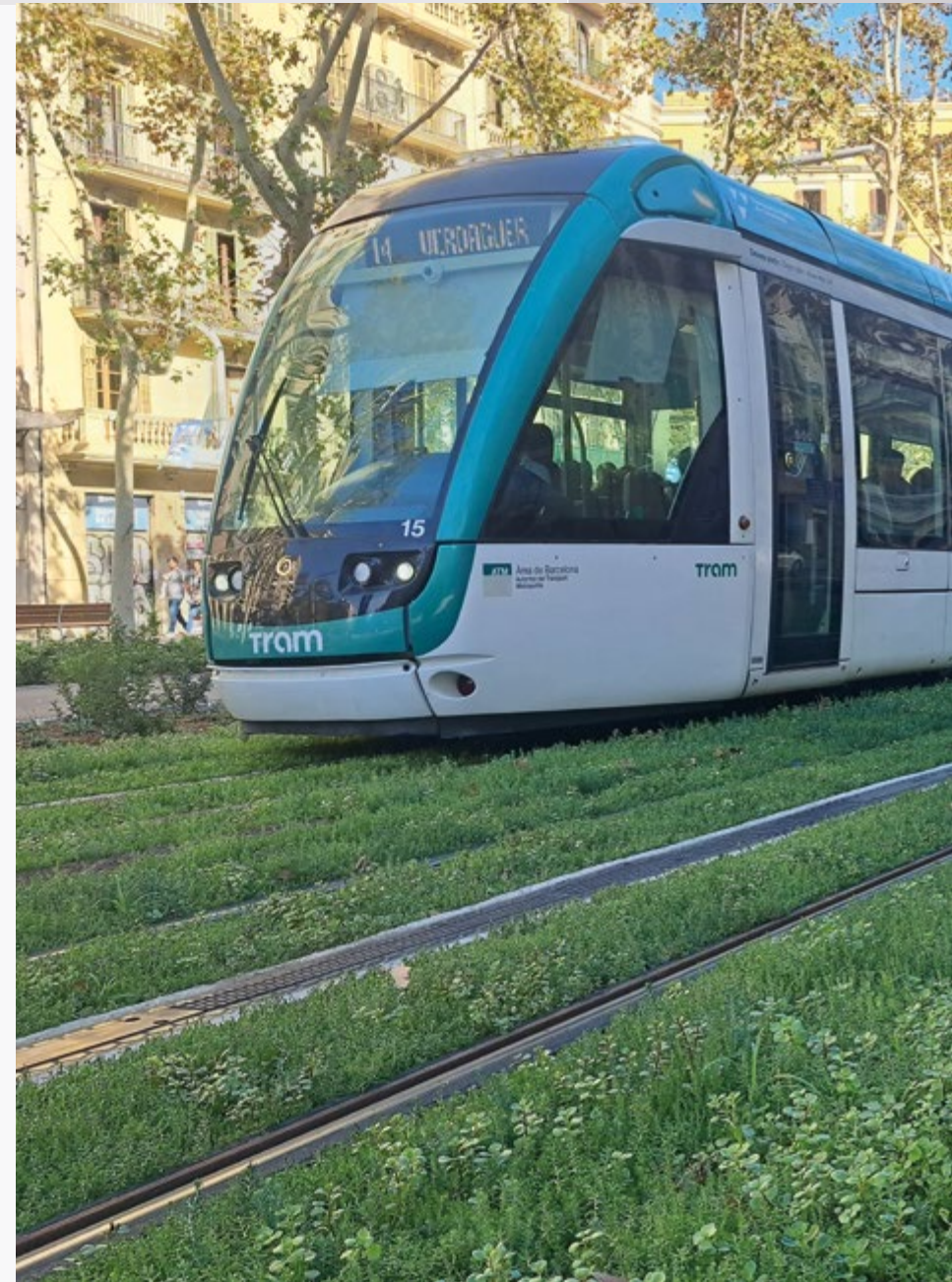
Completion of the Glòries - Verdaguer section of the tram in Barcelona (Spain).
