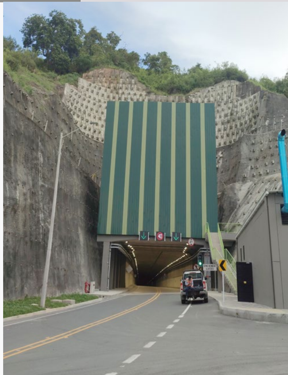
Tesalia Tunnel, the largest of its kind on the Pacific 3 Highway Connection (Colombia).
