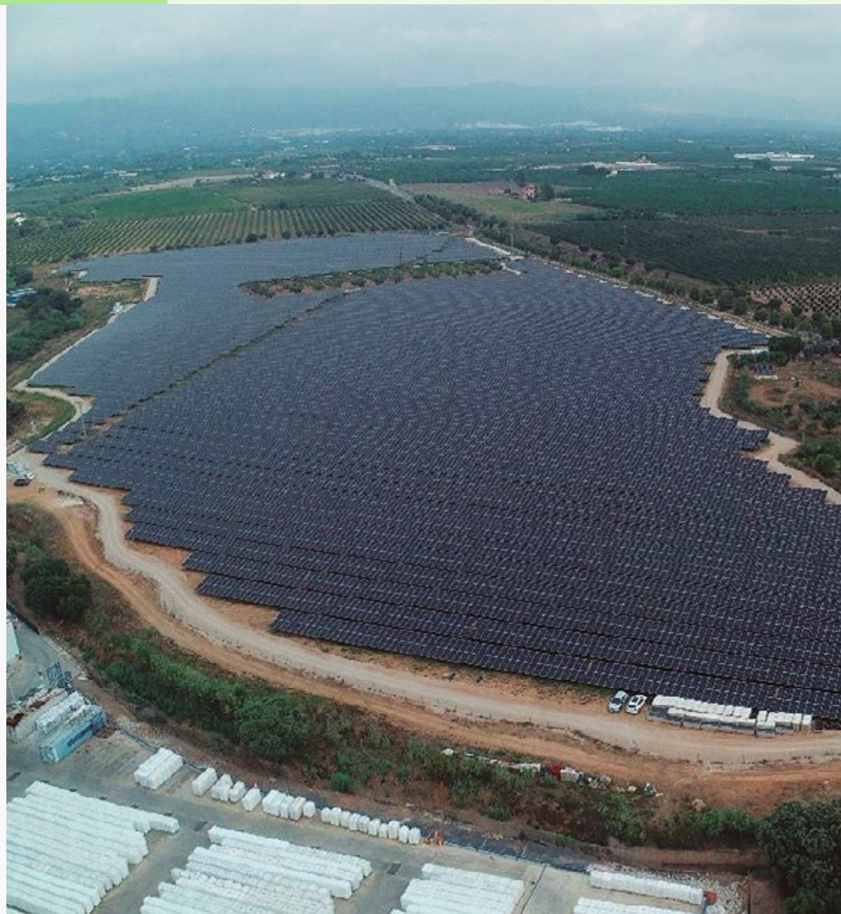
Photovoltaic plant in Constantí, Tarragona, with a capacity of 16.6 MWp (Spain). ▶
