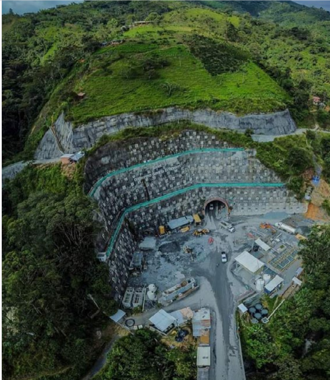
Electromechanical equipment, control systems, and radiocommunications for the ► Guillermo Gaviria Echeverri Tunnel project (Toyo Tunnel) and its access roads (Colombia).
