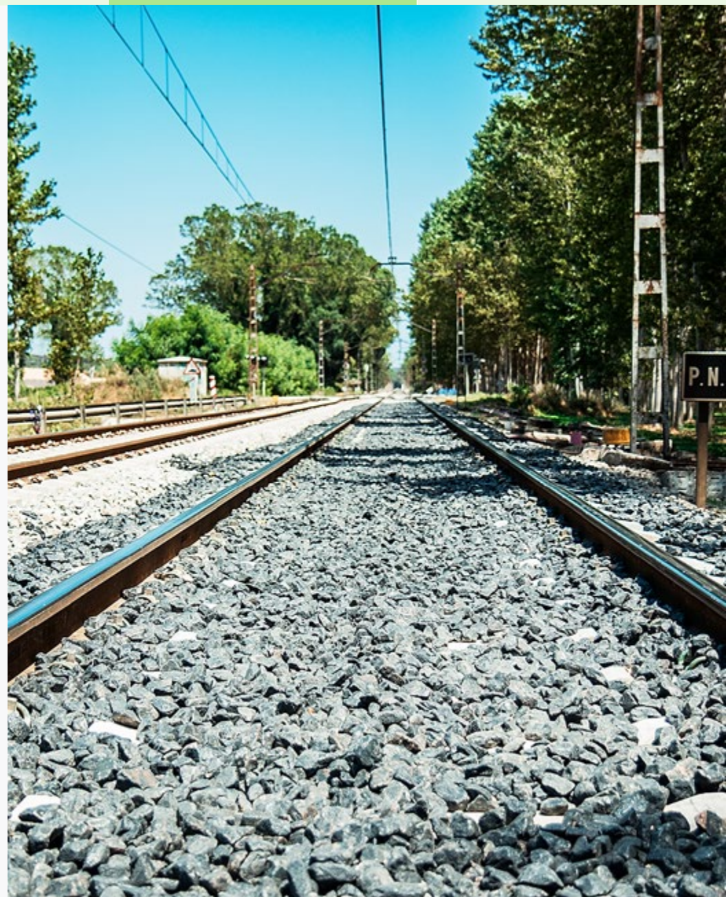
Pilot test of Neoballast on the railway segment between Sils and Maçanet de la Selva, Girona (Spain).
