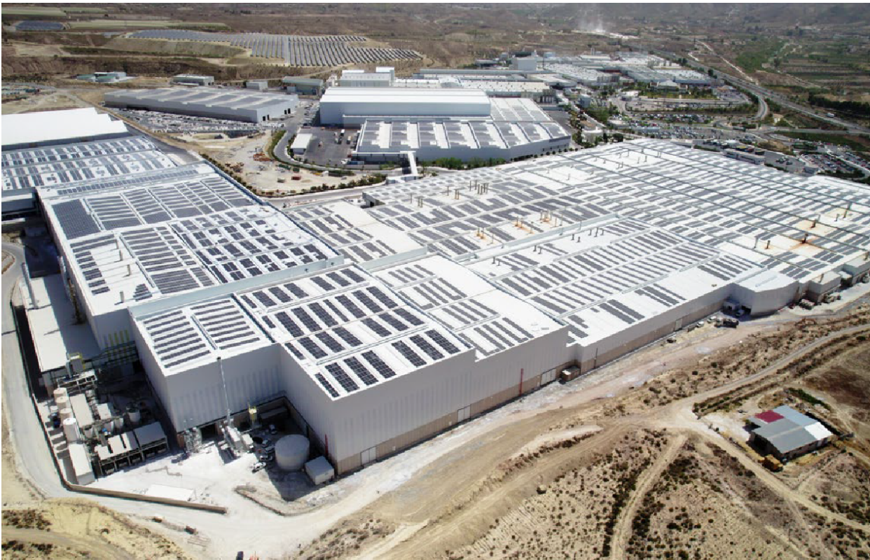
→ Photovoltaic installation at the Cosentino factory (Cantoria, Almería)
