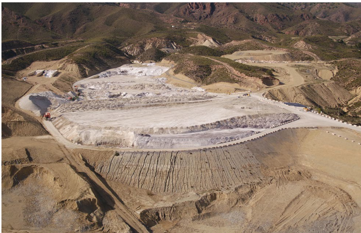
→ Cosentino's waste management plant (CoMA)
