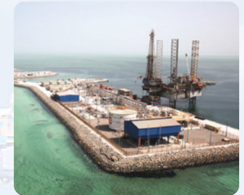
Hail Oil Field site terminal (Artificial island)
