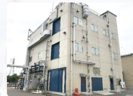
Exterior of EUV photoresist polymer production unit α3 (completed in 2022)
