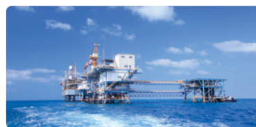
Cosmo Energy Exploration & Production Central Facilities Platform (CFP)
