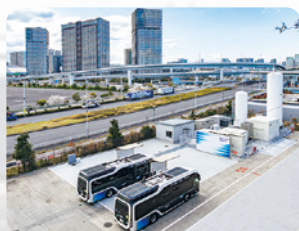
Iwatani Cosmo Hydrogen Station Ariake Bus Depot
