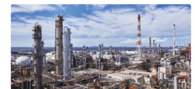
Maruzen Petrochemical Chiba Plant
