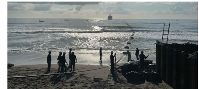
A landing station in Maruyama raising a cable
