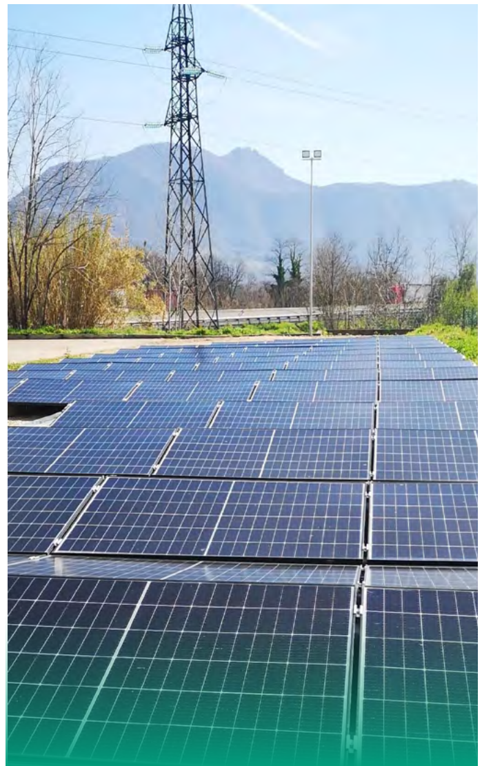
Solar panels at the Caserta plant, Antolin Italy.
