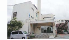
Iino Manufacturing Co., Ltd. Headquarters and the Omiya Plant (at the time)
