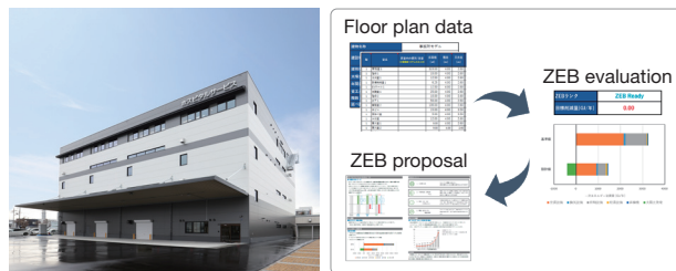
New head office of Hospital Service Co., Ltd. (Kyoto Prefecture): Office building and warehouse that meet the ZEB standard
