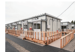
Slope used on approach
