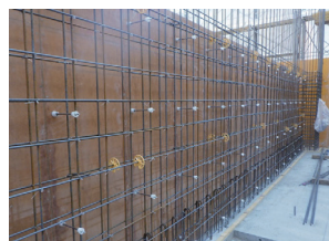
Base material is plywood made of particleboards recycled from construction scrap and 100% Japanese domestic timber.
