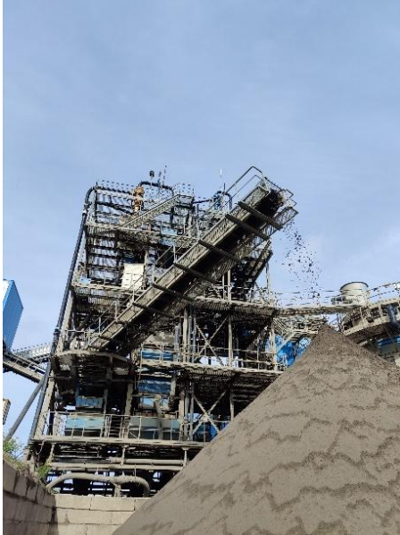
Washing installation BIOTERRA NV
