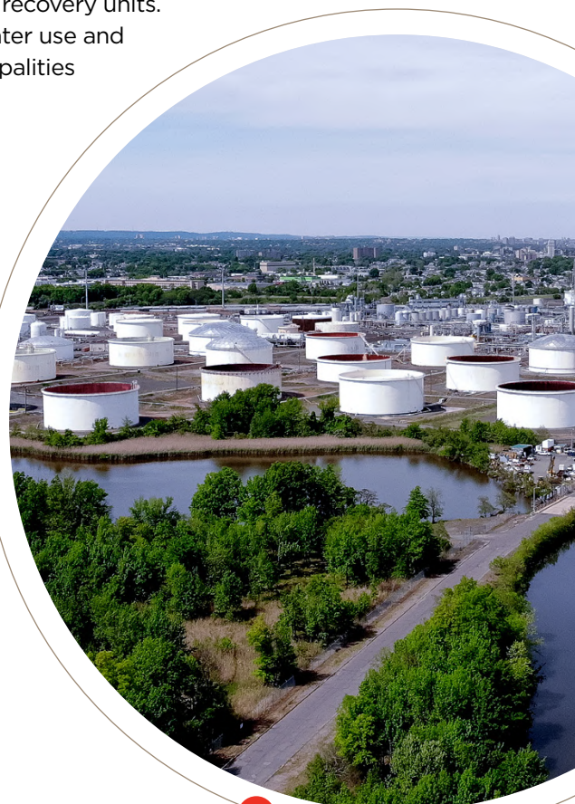
Bayway Refinery LINDEN, NJ
