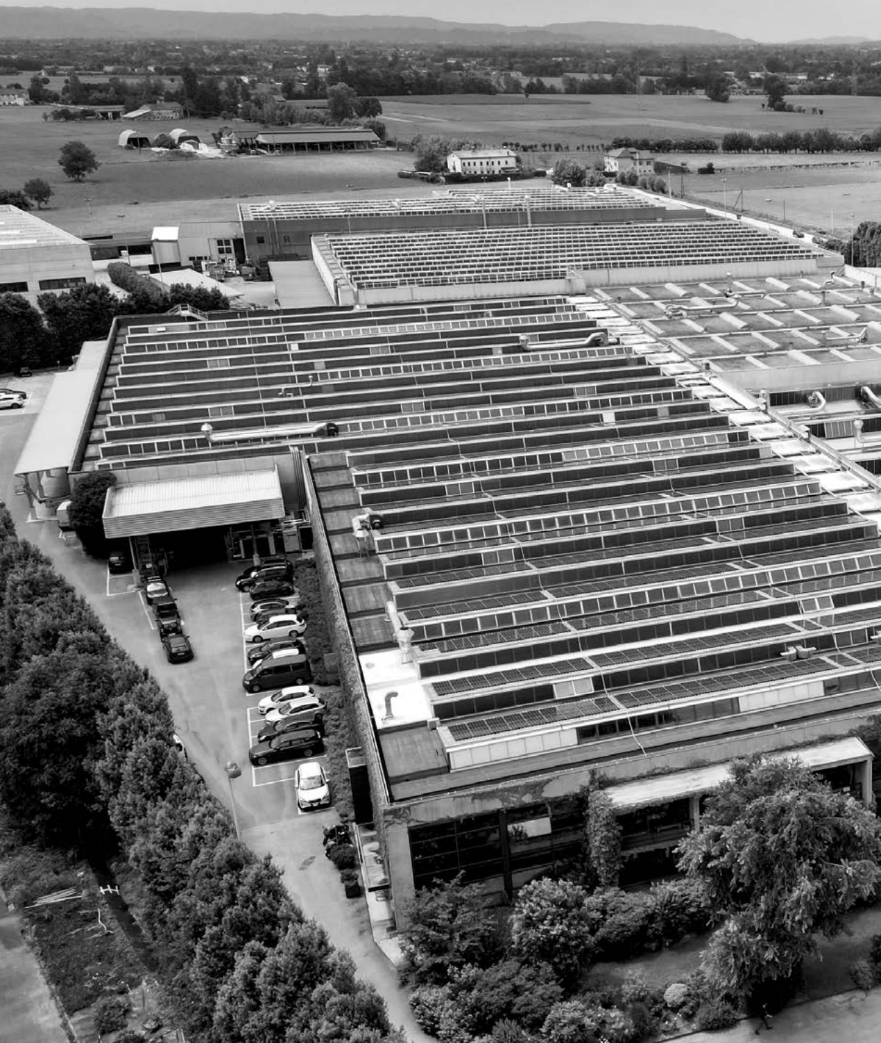
Solar panels on the roof of the Pozzoleone HQ, Italy—source: company archive
