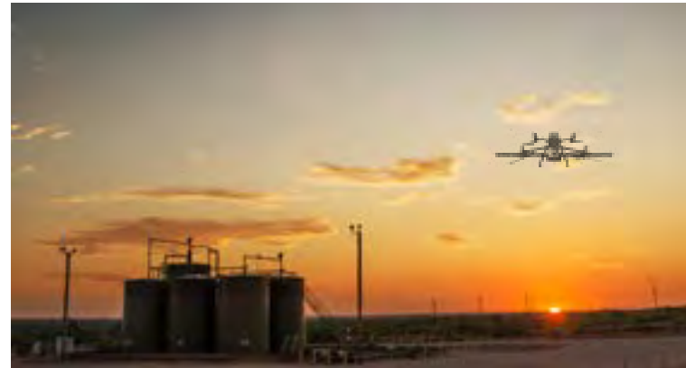
Drones that monitor our operations can help improve safety for our people in the field. Devon uses drones to inspect rigs and derricks for leaks and safety hazards, and to inspect long flowlines for leaks and pressure incidents. We prepared for the future of using drones for both safety and environmental applications by securing the first nationwide FAA waiver to use drones for commercial operations.
