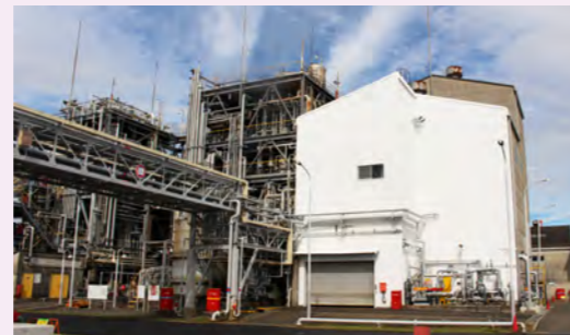
New dissolution and separation recycling facility
