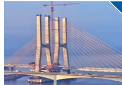
Zuari Bridge (Package II)
