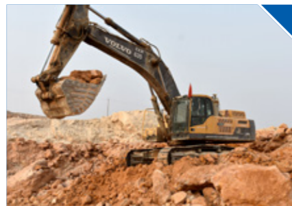
Nigahi OCP III (OB Removal Project)
