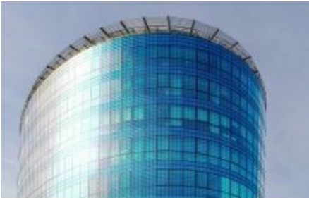
Installed on walls (provided by NEDO)
