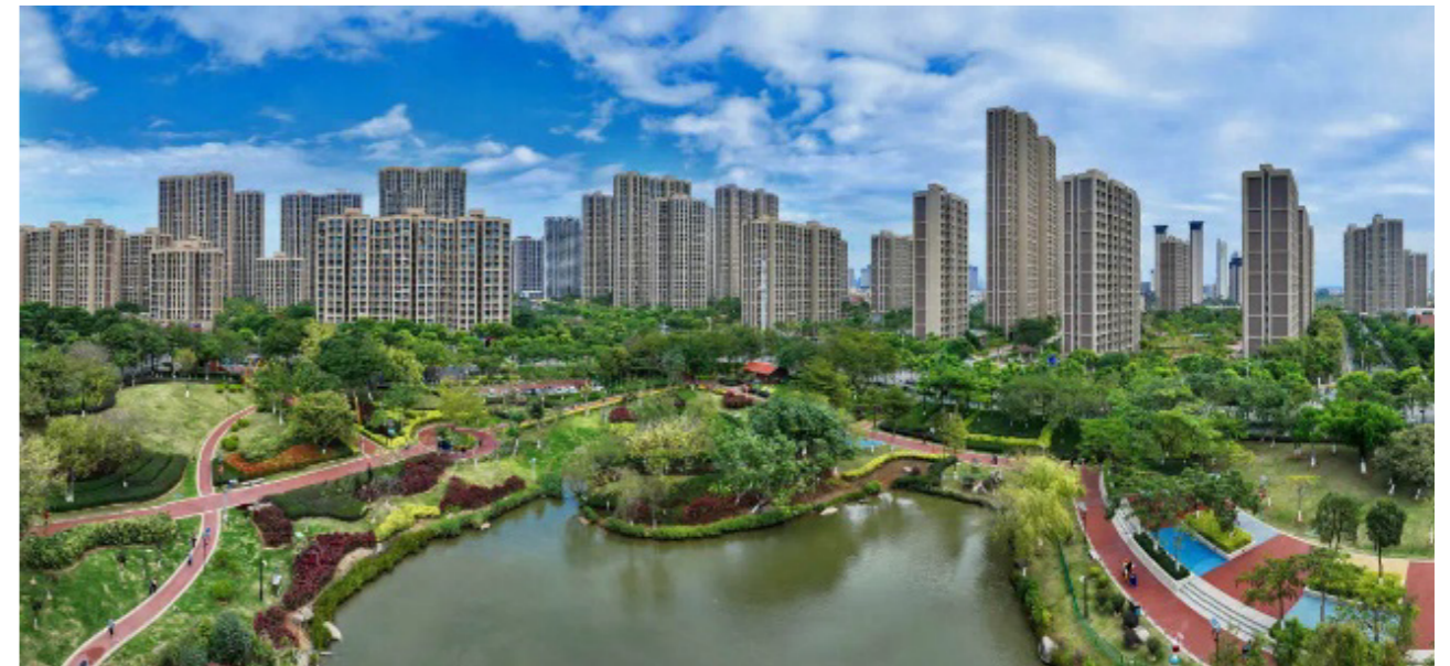
Affordable Housing Project in Xiamen Yangtang Residential Area
