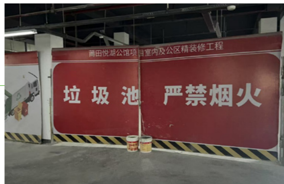
Collection Pit for Construction Waste
