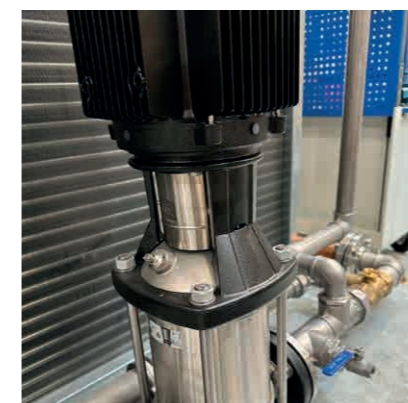
Power module and components for electrolyzer test bench
