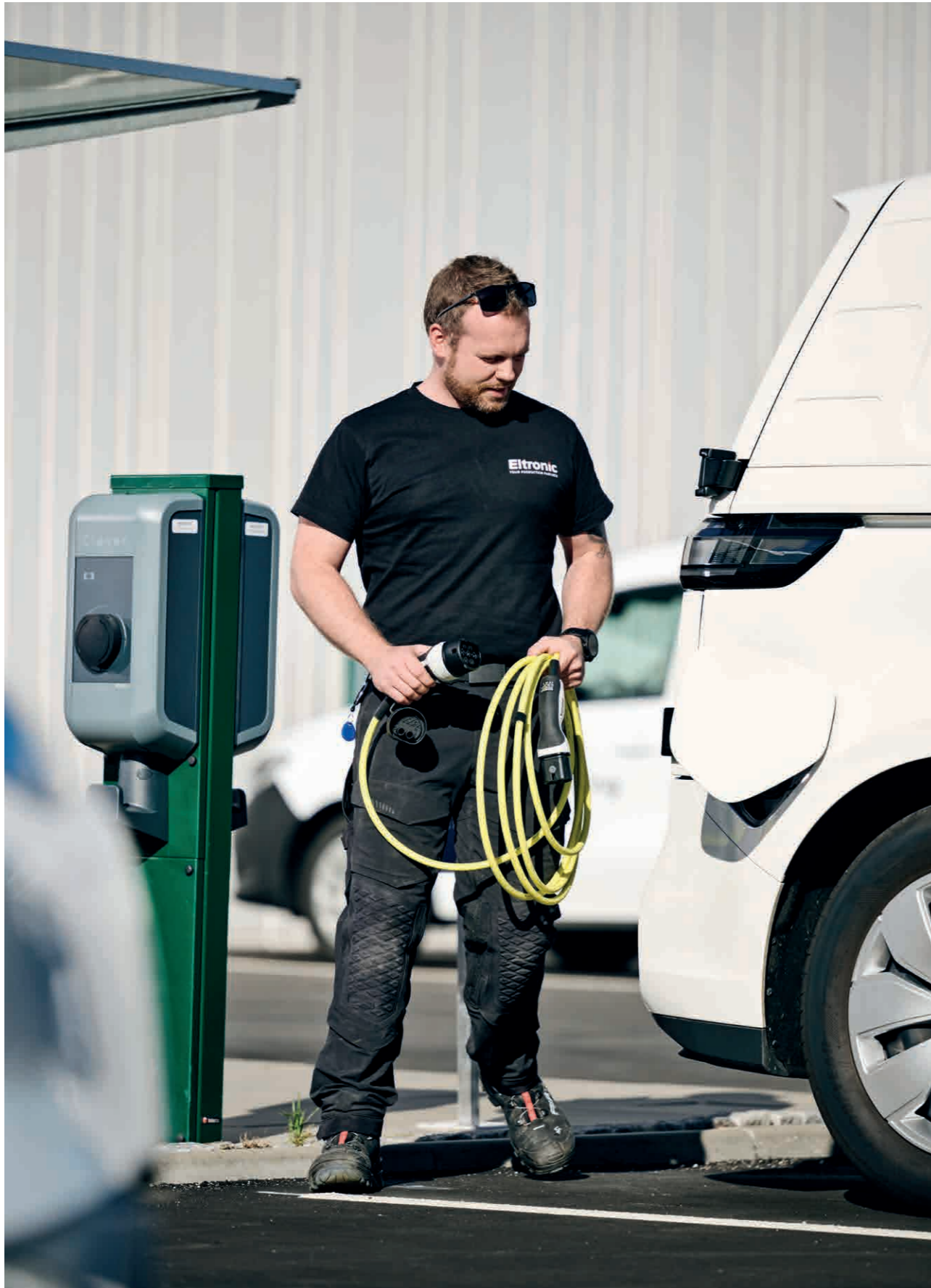
Morten Jensen, Electrical Service Technician, Eltronic A/S
