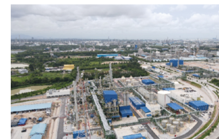
Aerial view of the new plant
