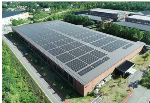
FANUC Headquarters (Reliability Evaluation Building)
