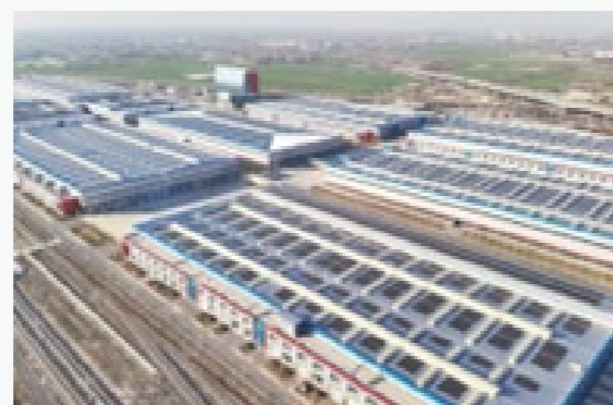
HBJC 6MW Distributed Photovoltaic Power Generation Project
