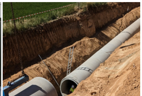
Prefabricated elements for sewerage pipelines of mixed sections, deployed on the sewerage and wastewater treatment works in Montijo-Puebla de la Calzada (Badajoz)
