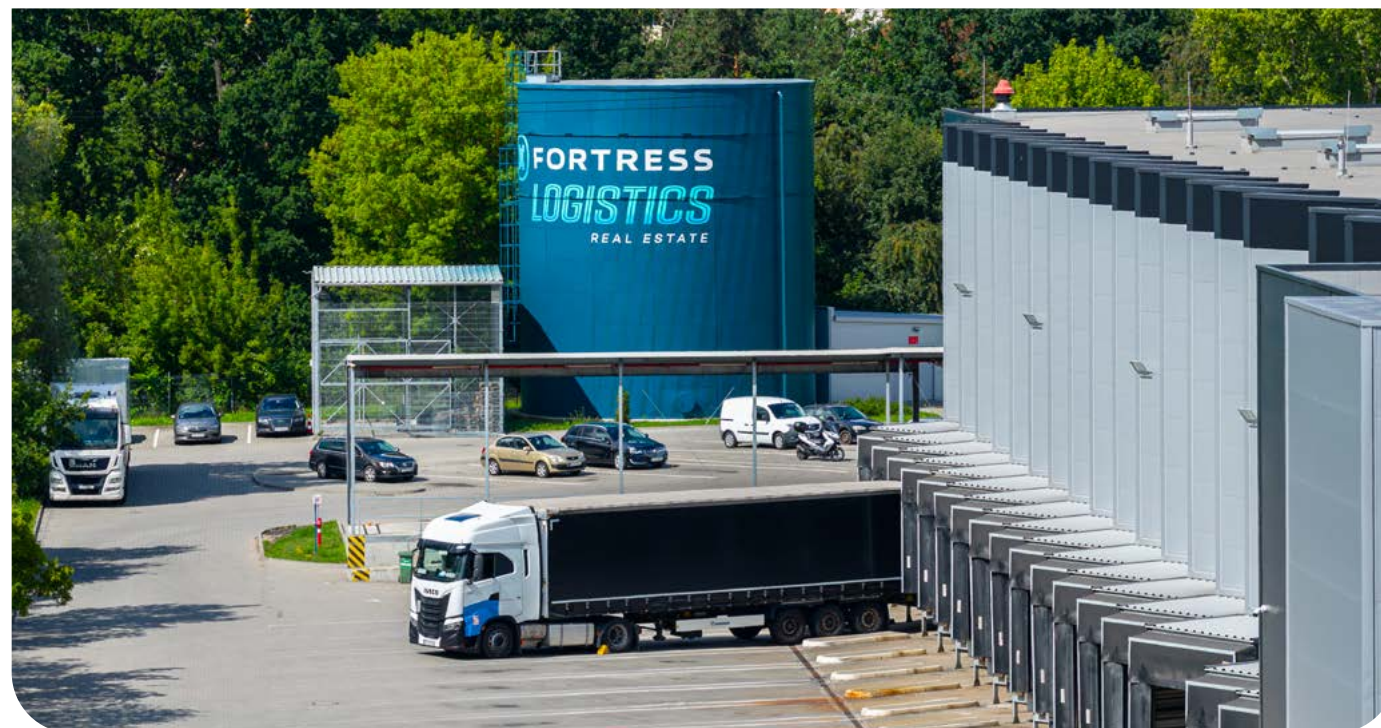
Water tank at Bydgoszcz Logistics Park
