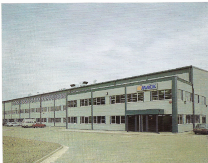
The new Fresh Produce Centre at Paddock Wood
